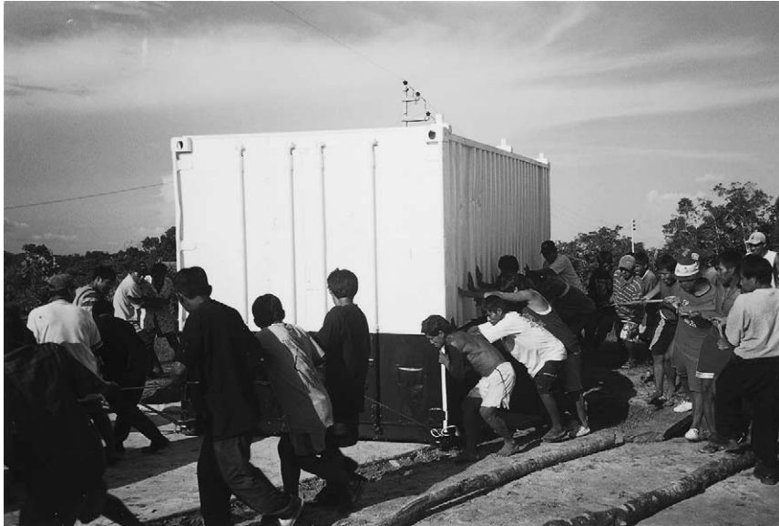
Fig. 6. Villagers provide manual labor in the final placing of one of the equipment housings.
